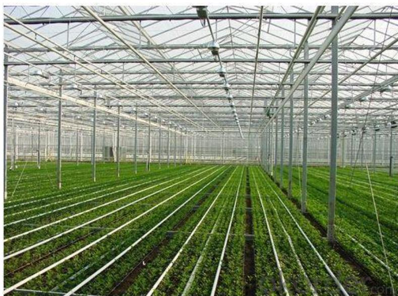
Slika 24. Plastenik s aluminijskom konstrukcijom ([https://www.okorder.com/p/thermal-screen-hdpe-with-aluminium-for-energy-saving\\_588502.html](https://www.okorder.com/p/thermal-screen-hdpe-with-aluminium-for-energy-saving_588502.html))
