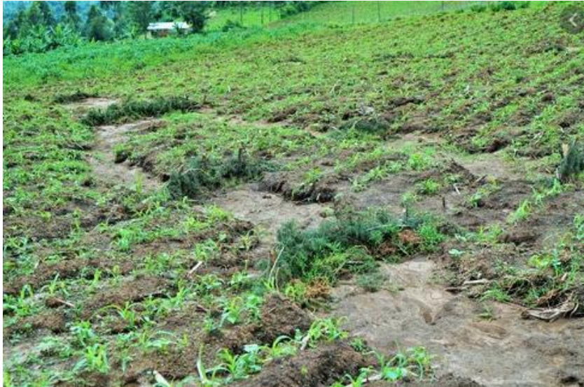
Slika 15. Posljedice vodene erozije (Izvor: http://mamase.org/news/soil-erosion-control-and-monitoring-interventions/ )
