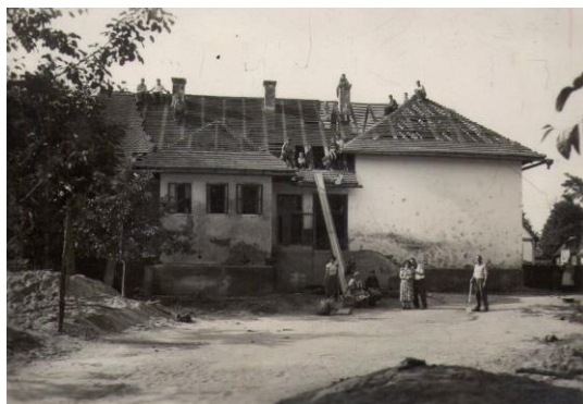
Sl. 12. Rušenje stare i nadogradnja nove školske zgrade izvor: https://www.facebook.com/banovajarugainfo/photos/a.267888740030706/268477399971840/?type=3&theater
